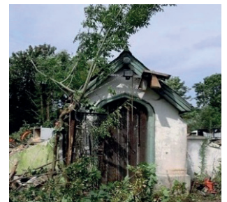
The chapel porch, shortly before its demolition.
